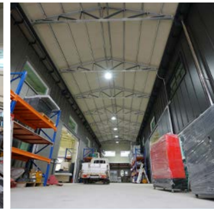
Inspection, assembly building
